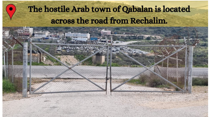
An upgraded new gate will enable Rechalim to efficiently monitor their surrounding & save lives!
