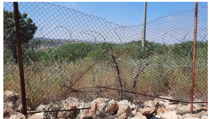
Salit's security fence is not an effective deterrent. You can help protect lives with additional surveillance cameras!
